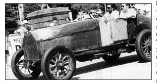
Detroit Model F "30" that had been fitted with two, in-line, four-cylinder engines. The engines were Chalmers "30" types, one a 1909 and the other of 1910 vintage. Conversion to dual-four operation was accomplished in 1916. This included some non-Chalmers items like the roadster body. Modifications to the stock Chalmers chassis accommodated the mounting of the second engine and the wheelbase remained unchanged at 110 inches. The addition of a second engine resulted in higher torque, slower
